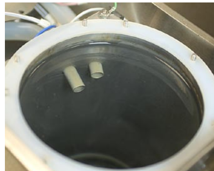
Water tank with Scale-Pro in use.*
